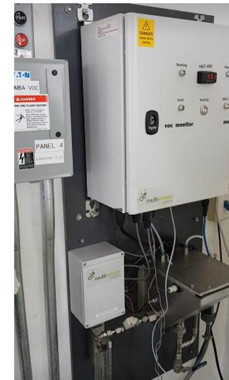
**Photo showing the MS1200 installed in the Pump Station. The unit is connected to a SCADA system (Ethernet) using the Profibus Protocol (TCP / IP), which records the data and, in case of an accident, activates the alarms that shut off the suction pumps.**
